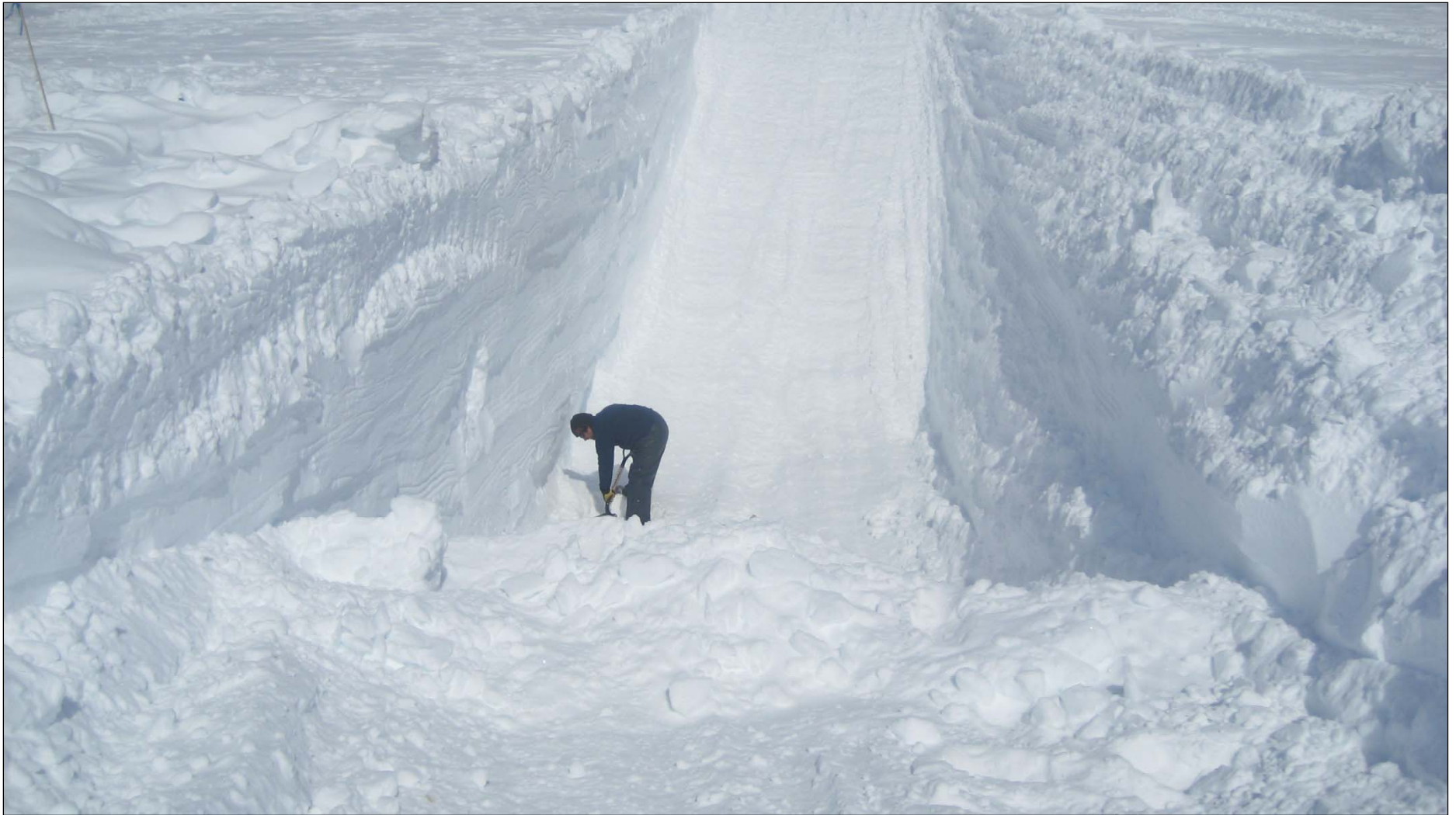
Trench in approximately four metres of snow covering the CH-1 kimberlite outcrop, May 12, 2009. Trench excavated by Bombardier Sno-Cat.
